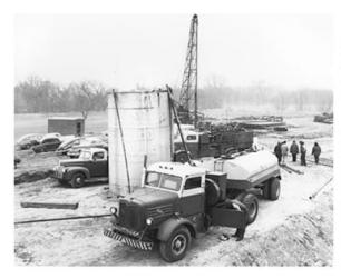
As shown in this historic photograph, the first hydraulic fracture treatment was performed by Halliburton under license to Stanolind Oil Company on March 17, 1949, east of Duncan, Ok. Hydraulic fracturing has since allowed commercial hydrocarbon recovery from more than 1 million wells that could not have produced economically, and that number grows by the day with nearly every U.S. gas well and the majority of all U.S. oil wells now being hydraulically fractured.
